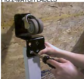
FIG.3-BOLT CASTOR TO THE BASEFRAME
